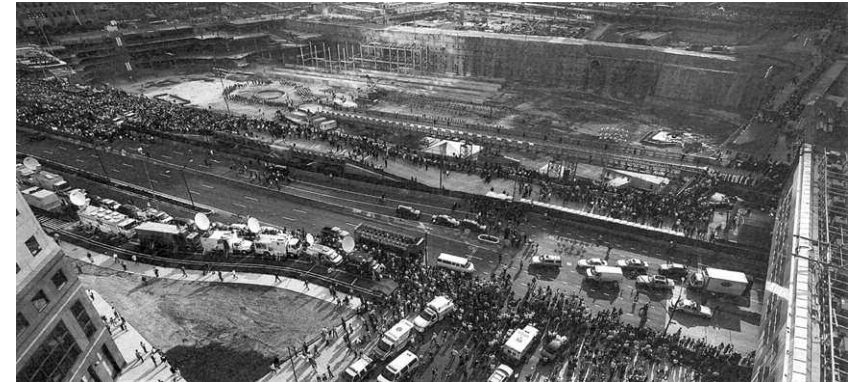
Fig. 20: Luc Delahaye, 11 September Memorial , 2002. Courtesy Luc Delahaye.
