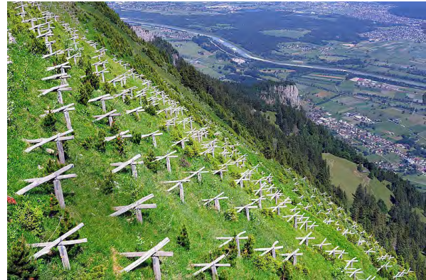
Fig. 12 | Lowinenschutz und Hangaufforstung , Walter Frehner, avalanche barriers lining up along the mountain slope.
