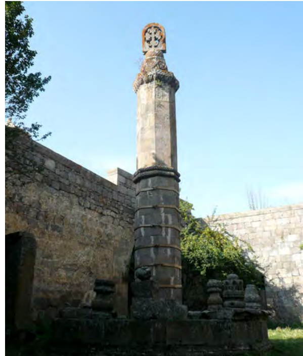
Fig. 9 | Tatev Gazavan . In the Tatev Monastery in Armenia, the resident monks constructed an eight-meter high prosthetic sense-extension as a response to a devastating earthquake. Erected in 904, the Gavazan obelisk expanded the monks' collective bodily capacity to detect seismic activity, warning them by tilting back and forth when slight seismic oscillations shook the ground. The hinged connection allowed the twelve segments of the octahedral structure to swing like a pendulum, turning back to its original position when danger was over. (Karakhanian; Abgaryan 2004) The researcher Vazgen Gevorgyan suspects an alternative function of the Gavazan in the form of a celestial compass. Aligned with the Orion belt, it served the monks as a prosthetic astronomical instrument for conducting time calculations, such as the duration of a year (Avetisyan 2018)
